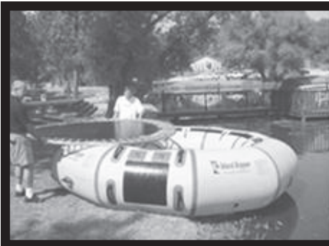
Lift completed frame on to tube
